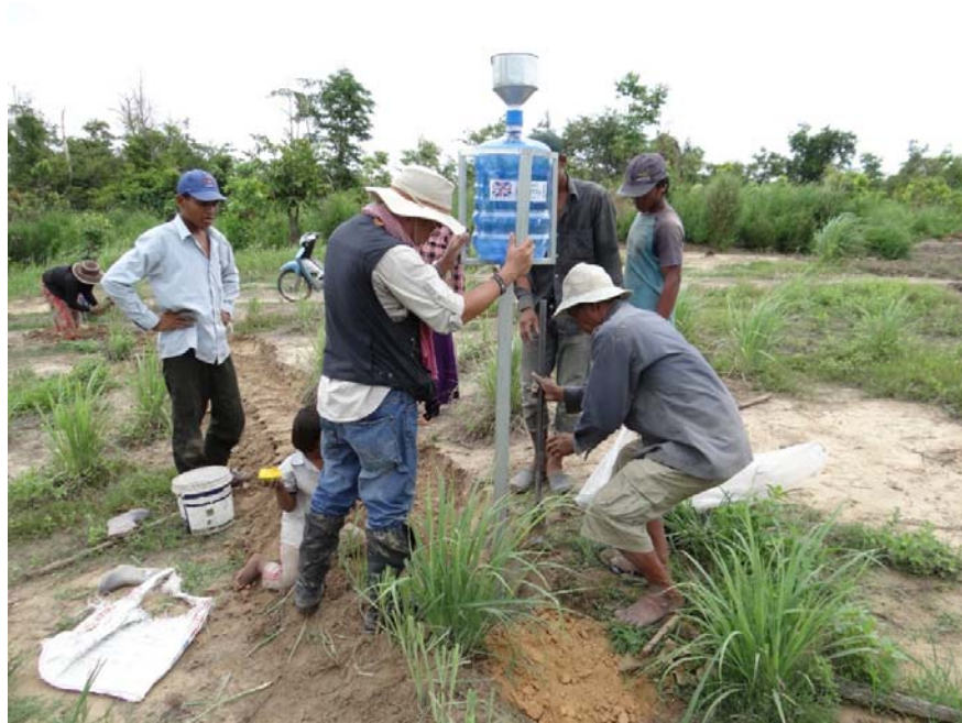
Photo 16. Installation of the rainwater collector
